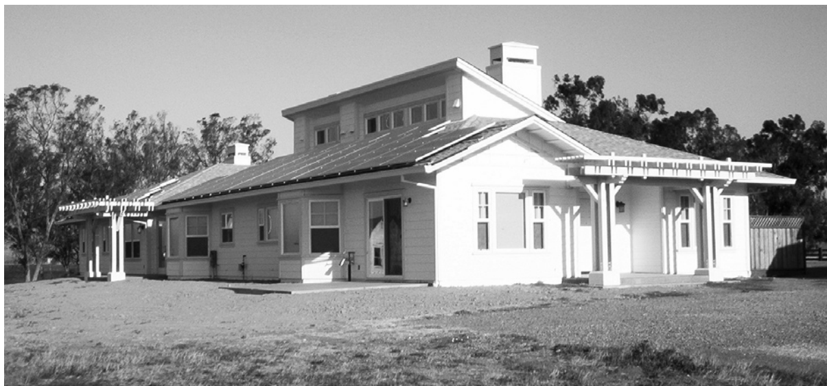
Solar panels contribute to the Center's off-the-grid energy needs
